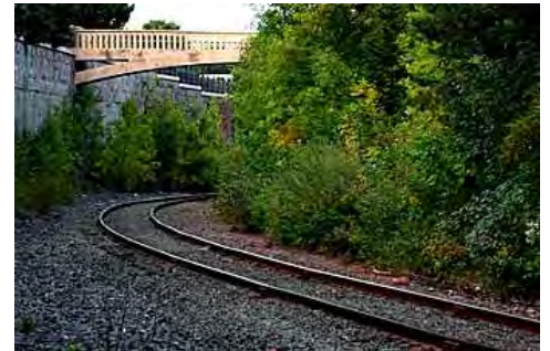
3rd Place Dick Anderson Curving Track
